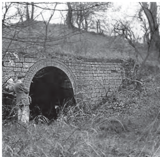
The western portal of Norwood tunnel in 1959.
